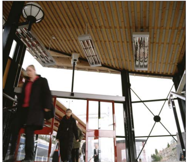
This train station outside Stockholm is heated by industrial infrared heaters. A regulator with timer allow waiting passengers to increase the heat when it is particularly cold.
