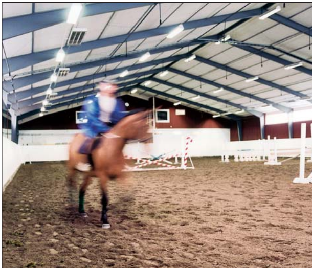
Radiant heating heats people directly without warming the surrounding air. The operative temperature, i.e. the temperature a person senses, is therefore a little higher than the actual temperature. Every degree reduction will save approximately 5% of the energy consumed!
