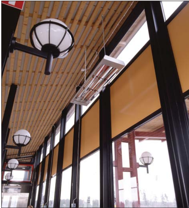
This train station outside Stockholm is heated by industrial infrared heaters. A regulator with timer allow waiting passengers to increase the heat when it is particularly cold.
