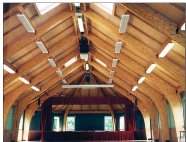
Radiant heaters provide flexibility. Buildings that are used on an irregular basis can be heated fast without a high energy consumption.
