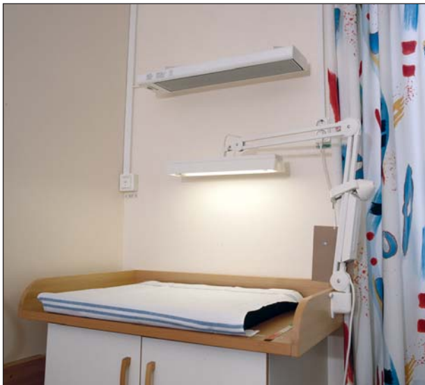
Elztrip make sure that the newborn babies are not cold at this maternity hospital outside Stockholm. Radiant heaters give a soft, hygienic and discreet zone heating. EZ100 heats silently, without air movements and with maintained air quality.
